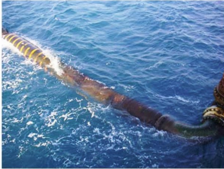
Floating Discharge Line
